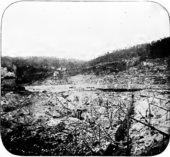
Foundation Masonry of New Croton Dam.
