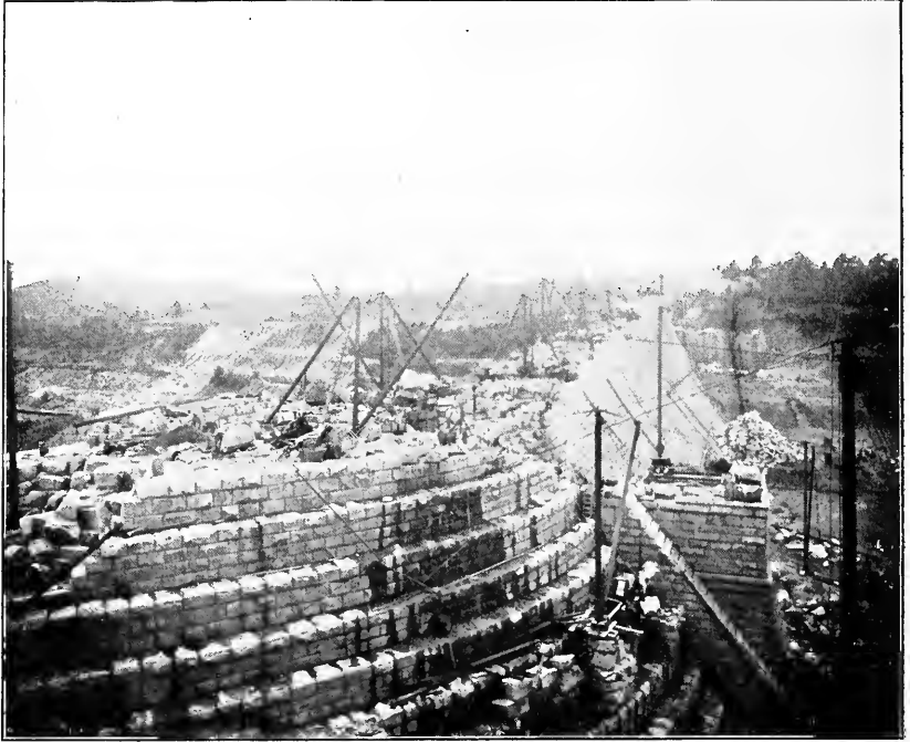
Progress View of Construction of New Croton Dam.
